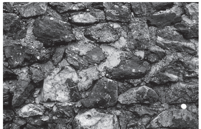
Figure 8. A rough wall made of angular blocks of veinstone and tourmalinized killas, Sandy Hill, near St. Austell. This veinstone probably came from Charlestown United mine, which is only a few hundred metres away. The tourmalinized killas may have come from stream tin workings in the Sandy valley.
