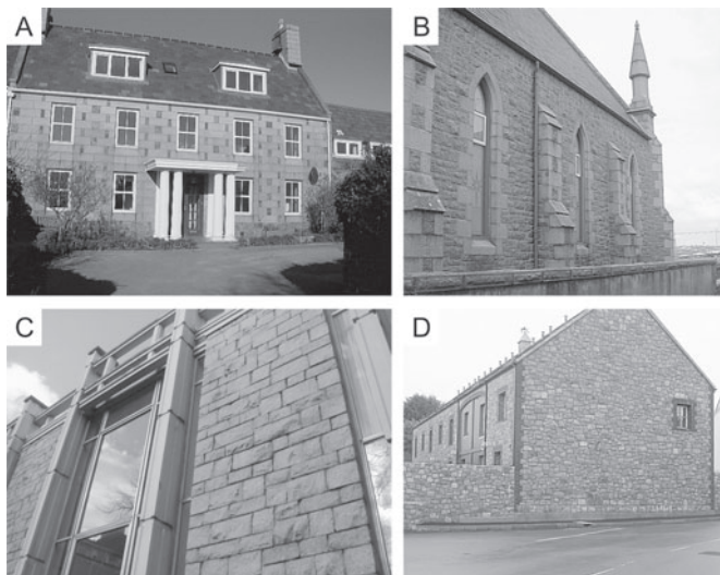
Figure 5. (A) The regularity of the ashlars used for this house front is typical of the nineteenth century but what is much rarer is the geometrical interspersing of the granite with diorite. (B) Granite is a very difficult rock to sculpt and, even with nineteenth century techniques it was rare to find much detail. More typical are the Victorian gothic shapes shown here from a local chapel at St. Aubin. (C) During the latter 1960s and early 1970s, Ronez Quarries worked the L'Etacq Quarry SE using a thermal lance and cut the blocks produced into regular sawn and split ashlars. It was hoped that a block layer could be used to set them but the end result was better if a stone mason was employed to trim the quarry pieces. (D) In the last two to three decades many buildings, often those of commercial enterprises in the town, have used natural stone finishes but some are rather spoiled by the creation of large unrelieved surface areas.
