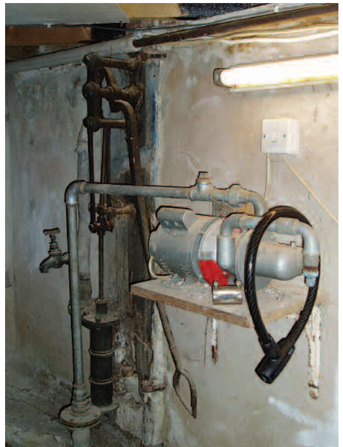
Figure 4. Old hand pump and modern electric pump above the spa well in the cellar of Nottingham Spa House, photographed in 2007.
