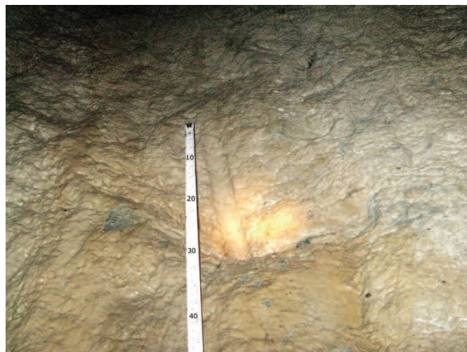
Figure 14. Flowstones coating vertical shaft walls and gunpowder blast shot hole. Decimetre spacing highlighted on tape measure. Photograph: Geoff Purcell.
