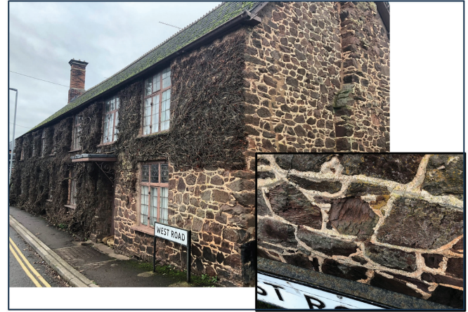
Figure 7. Typical building style exhibited in West Road with inset showing irregular arrangement of building stones.
