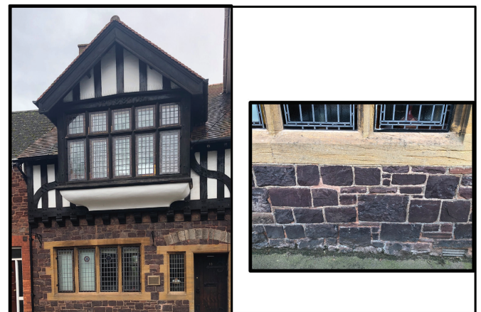
Figure 4. The most common building stones in Wiveliscombe: the Devonian Pickwell Down Sandstones, exhibited here in the Old Reading Rooms; inset shows regularly shaped blocks of ashlar. Note use of Ham Hill Stone for the surrounds of windows and the door.
