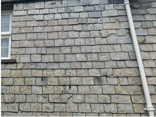
Figure 2. Morte Slates-cladding a west facing wall of one of the taller buildings of Wiveliscombe.
